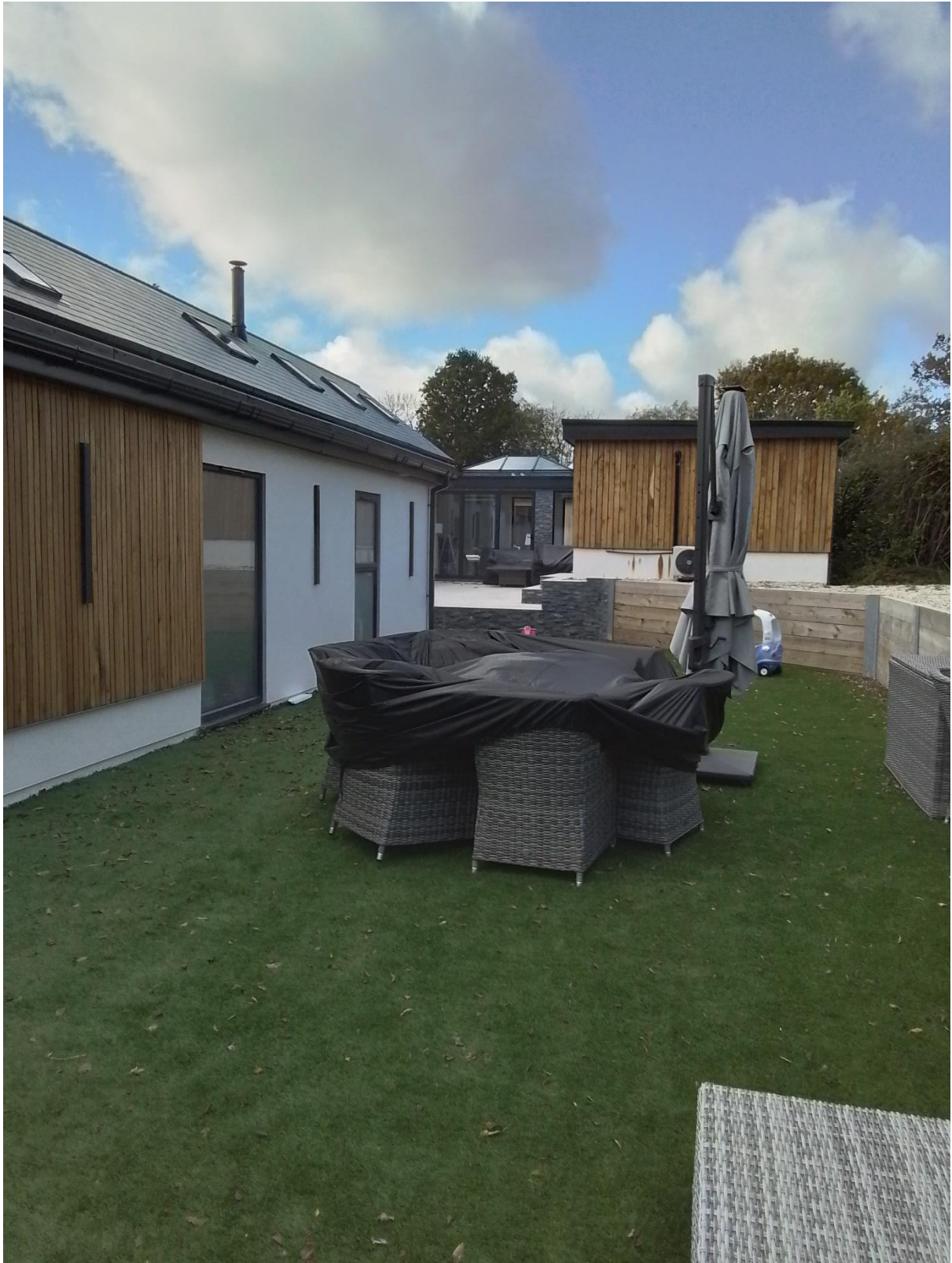
North elevation showing roof & retaining walls
