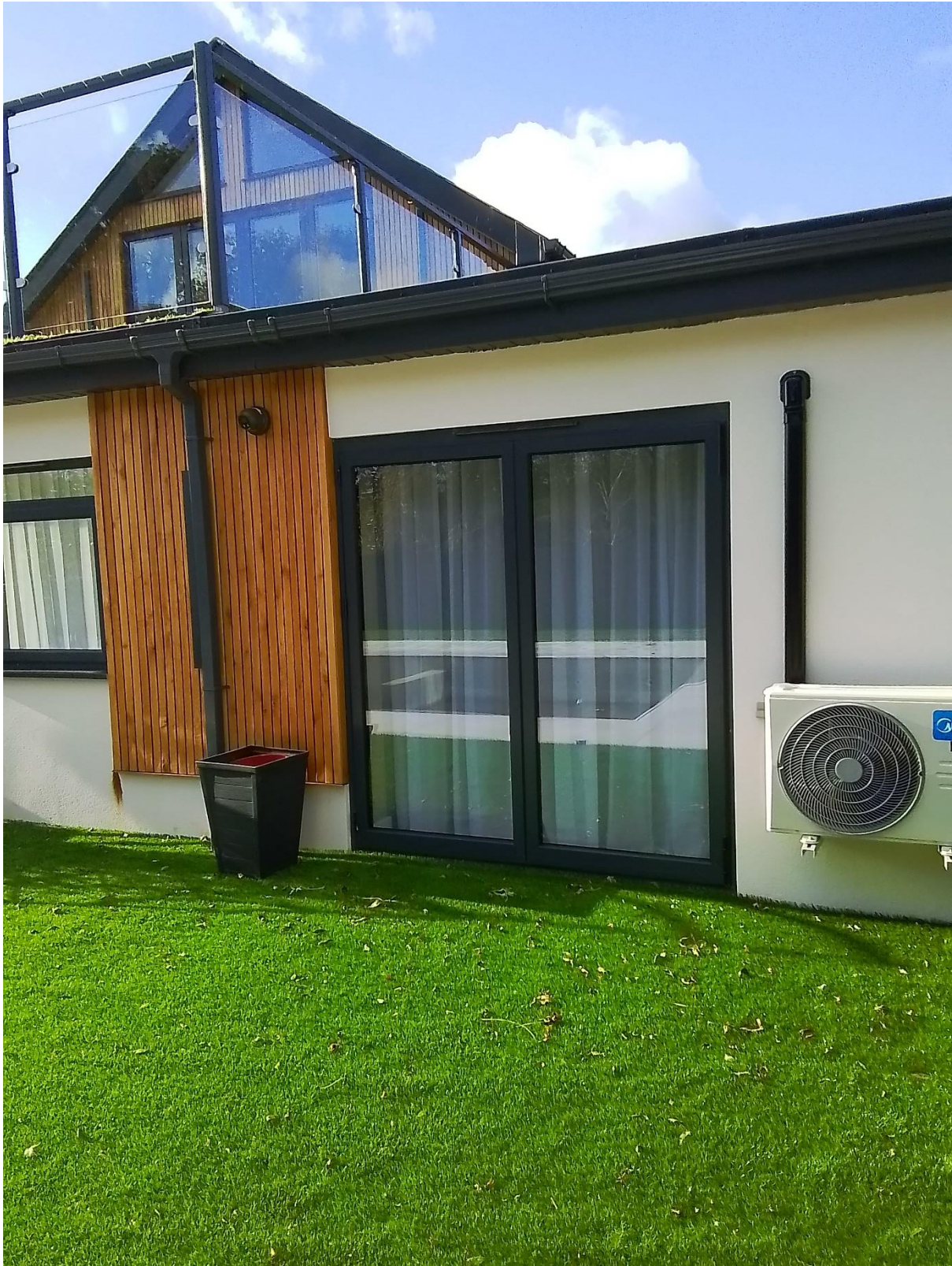
Eastern elevation with 1st floor extension
