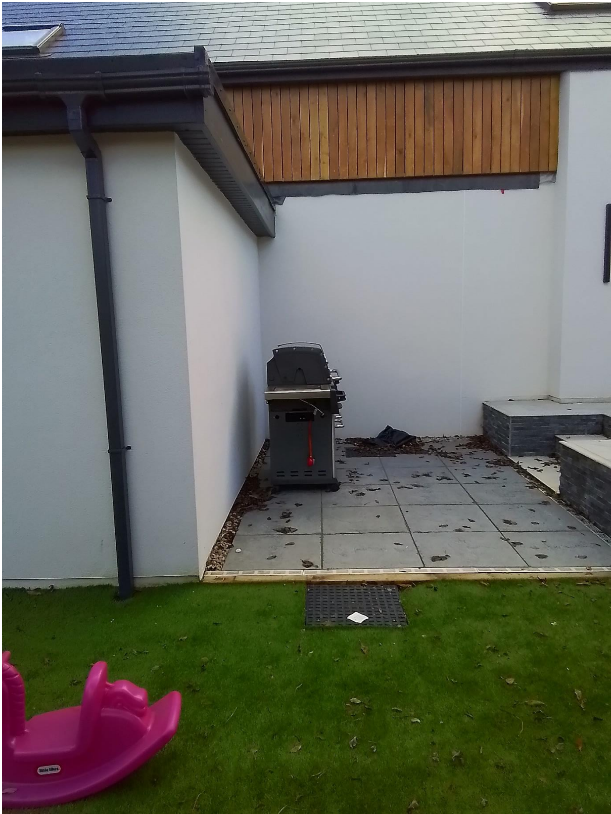
End of first floor wrap around extension looking S
